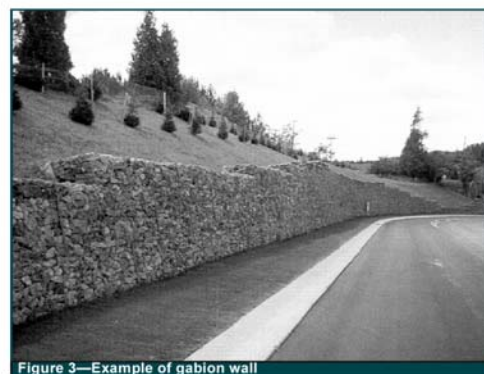
Figure 3—Example of gabion wall
